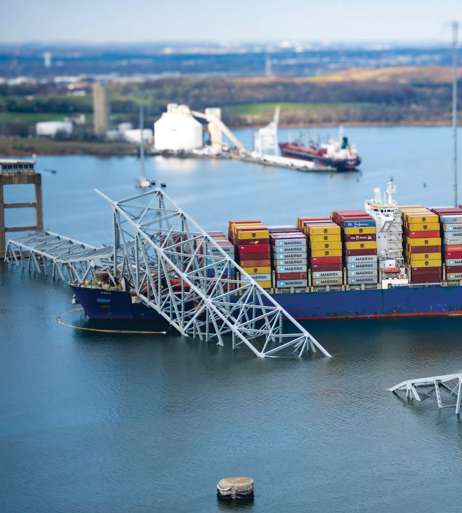
While leaving the Port of Baltimore in the early morning hours of March 26, 2024, the Singapore-flagged M/V Dali , a neo-Panamax container ship, lost power before striking a Francis Scott Key Bridge support, causing the bridge to collapse. Coast Guard photo by Petty Officer 1st Class Brandon Giles
